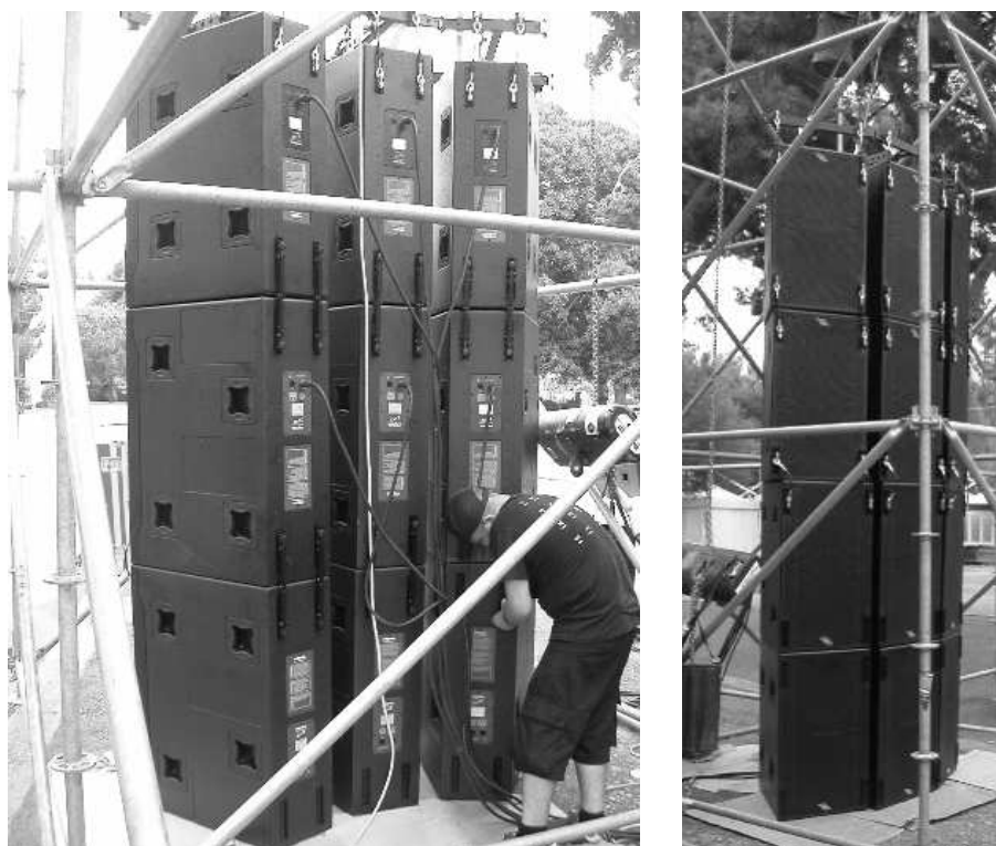
Figure 5.21: Array cabled and ready to be lifted
