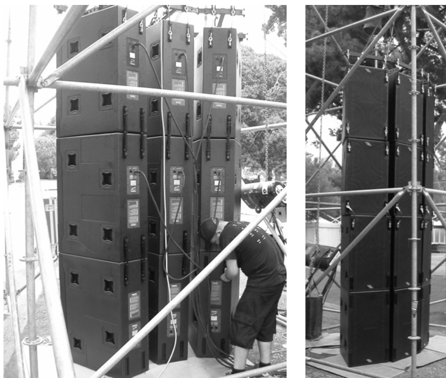
Figure 5.21: Array cabled and ready to be lifted
